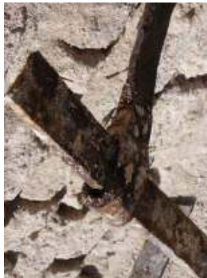
Figure 12: External end of transverse tie-rod
