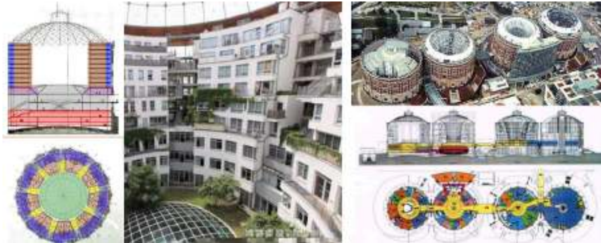
Figure 4: Division and multiplication systems. On the left, the interior of each gasometer is divided in several parts. On the right, the four Gasometers are connected with a new element to create a continuous area.
