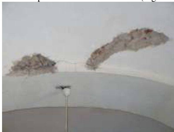
Figure 14: Cracks in the masonry vault and arch
