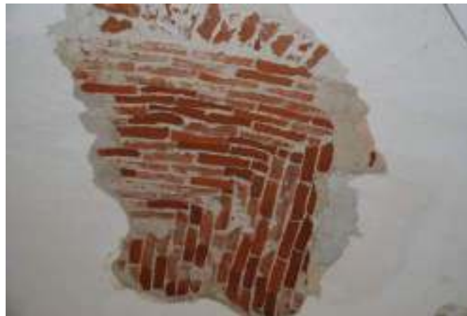
Figure 2: Swallow-tail technique of waving bricks for a Bohemian vault
