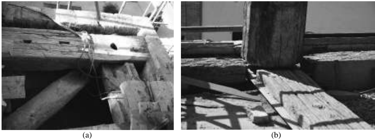
Figure 13: Floor ties between the columns: (a) corner, (b) strengthened with steel profiles
