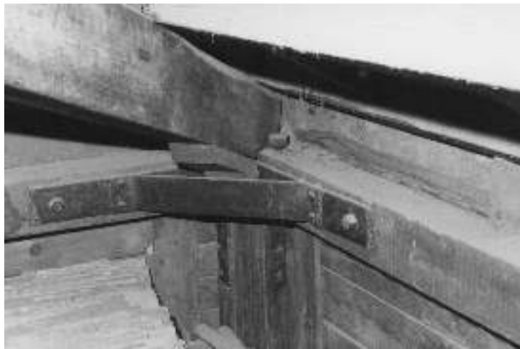
Figure 10: Metallic handmade elements to stiff and reinforce angle beams in the upper part of the structure. San Sperato House (Reggio Calabria); similari to the one of Cav. Ferruccio Gay at the beginning of ‘900.
