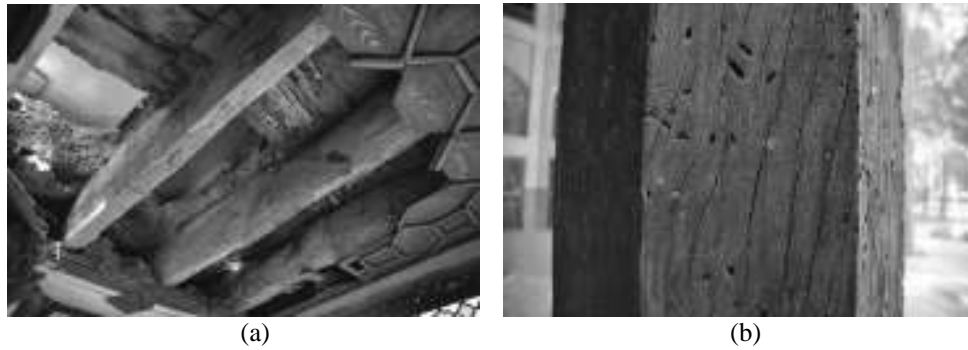
Figure 20: (a) Termite attack, Mosavver-al-Mulki house, Isfahan, eighteenth century A.D., (b) beetle holes, Hasht-Behesht building, Isfahan, 1897 A.D.
