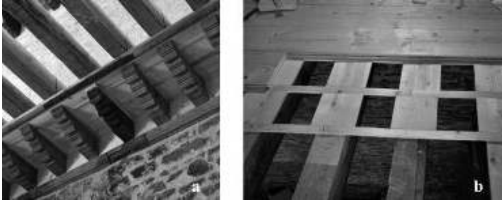
Figure 10. a. The in situ remaining original 12 th corbel and underlying cornice, with the new corbels and beams. The lower coffered ceiling between corbels and beams is already in place. Discernible is the original braid element, that was found reused in the Ottoman wing by chance. b. Constructing the coffered ceiling over the beams. The cantinelle running transversally to the beams are made of strips as original, whereas the ones parallel to the beams are made of planks projecting over the edges of the beams, ensuring full contact of floor boarding and beams. Note some tongue and groove boarding planks that have already been screwed into place
