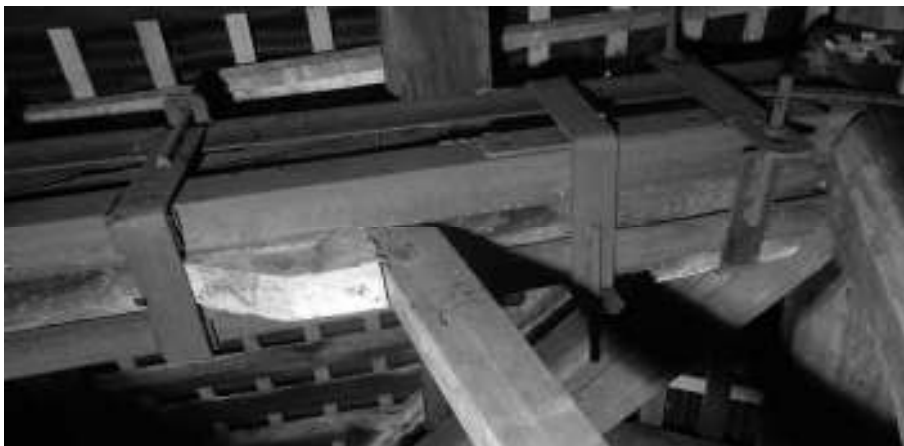
Figure 14: Strengthening system for the rafter of truss 5 (photo by M. Bosi, A. Cernuschi, E. Doria, P. Pilan).
