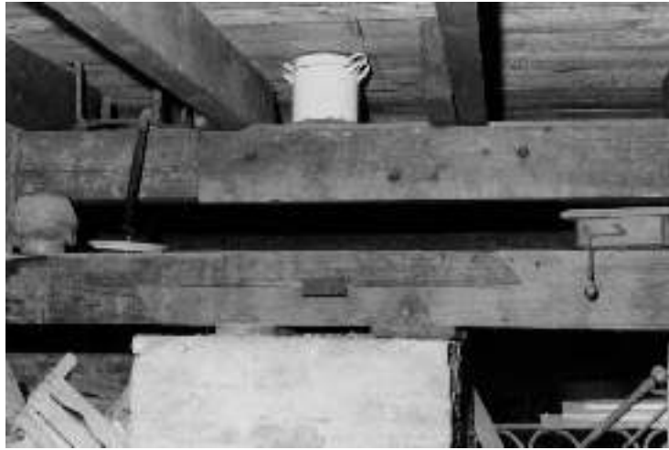
Figure 9: “stop-splayed scarf with key” joint that connect two sleeper in the foundation. San Sperato House (Reggio Calabria); similar to the one of Cav. Ferruccio Gay at the beginning of ‘900.
