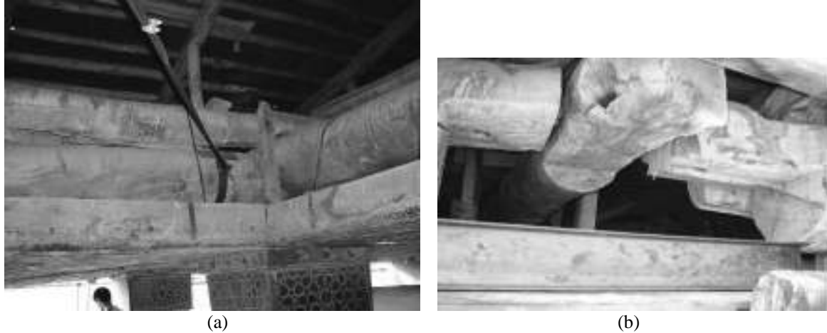
Figure 17: (a) Secondary beam over the main beam over the column with a steel cable lateral bracing attached to the main beam, (b) a steel profile for strengthening the wooden beam
