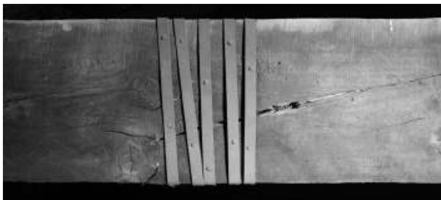
Figure 8: System used for the strengthening of the tie-beam of truss 5 (photo by E. Zamperini).
