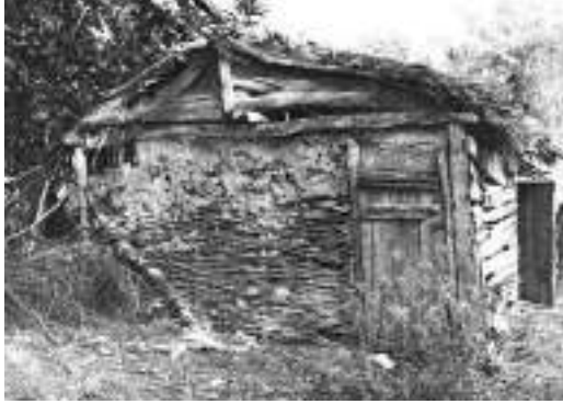
Figure 16: Interlaced twigs on a timber skeleton rural building (Yakar, J., Garson, J. L.)
