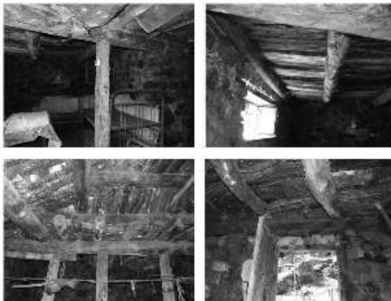
Figure 2: Photos of Tchatchkari dwellings. Medieval log and timber ceiling constructions.
