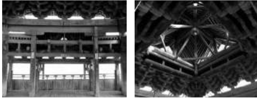
Figure 5: The columns, girders of the third floor and the bracket set on the top of Feiyun Pavilion
