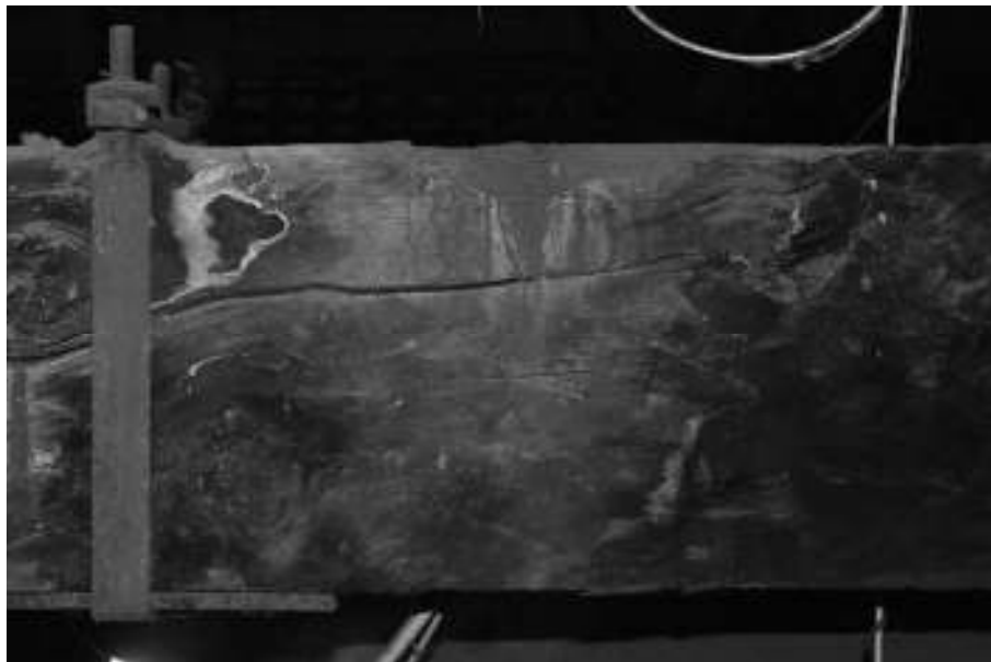
Figure 15: Incipient biotic decay phenomena in the tie-beam of truss 2 (photo by M. Canestrà, R. De Marco, R. Delogu, G. Godio).
