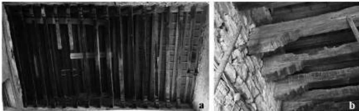
Figure 5. a. The second floor remains, underneath the modern roof. b. Closeup of some of the second-floor beams and corbels, before restoration began
