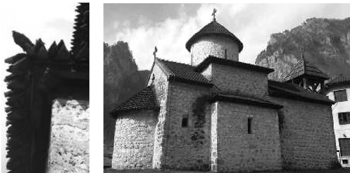
Figure 8: Details of roof cladding decay and rain water traces on walls of Monastery Dobrilovina
