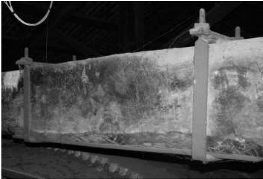
Figure 9: System used for the strengthening of the tie-beams of truss 2 and 4 (photo by E. Zamperini).
