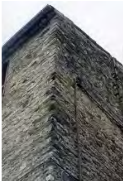
Fig. 4 Unit 396 showing good connection.
