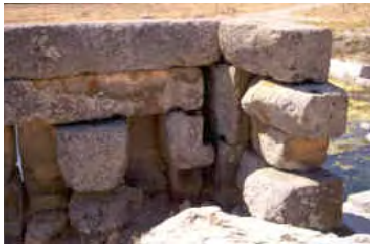
Figure 6. Detail of Blocks Prepared for Easy Handling
