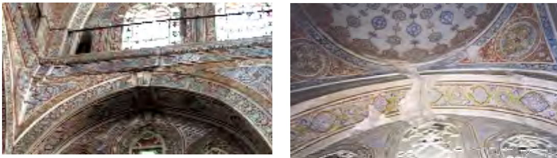
Figure 2 Damaged arches in the gallery level of the south wall
