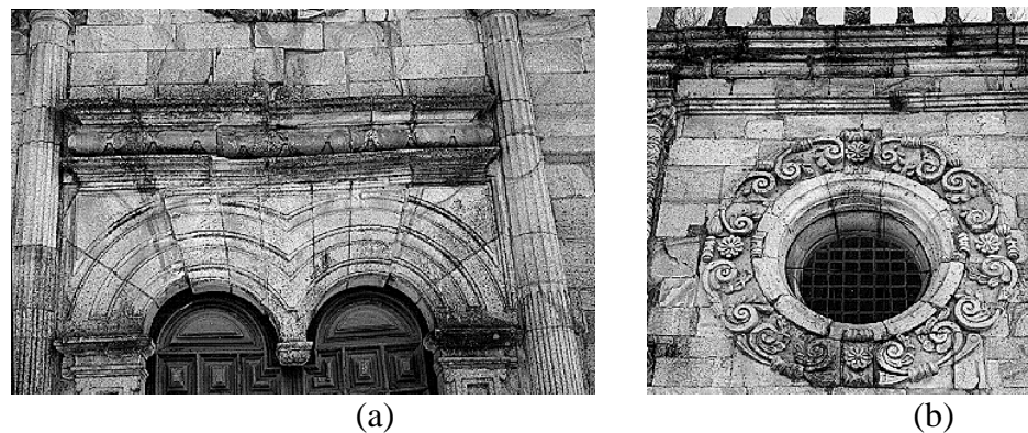
Figure 3 – Damage in the façade: (a) twin arch and (b) opening
