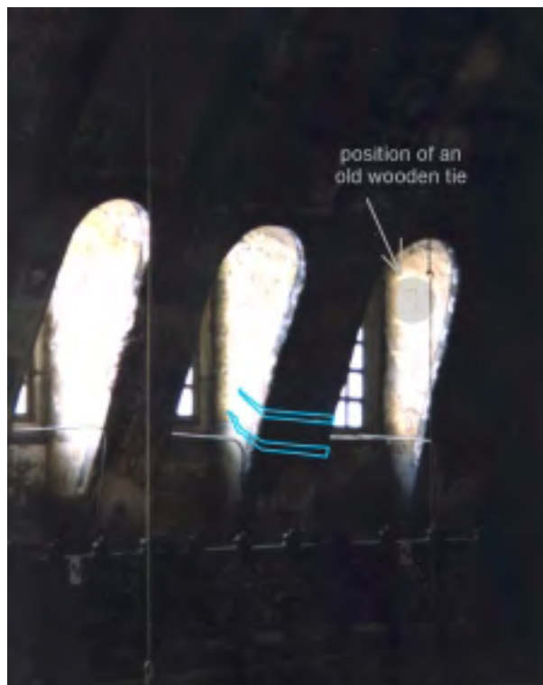
Figure 9. Photo of the windows at the base of the dome. The cracks on the ribs and the position of the old wooden ties are clearly shown.
