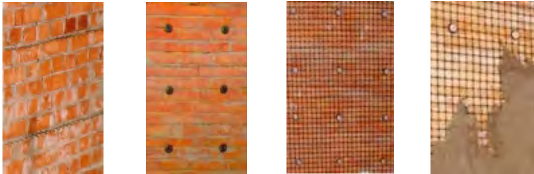
Figure 14 Horizontal and vertical reinforcement
