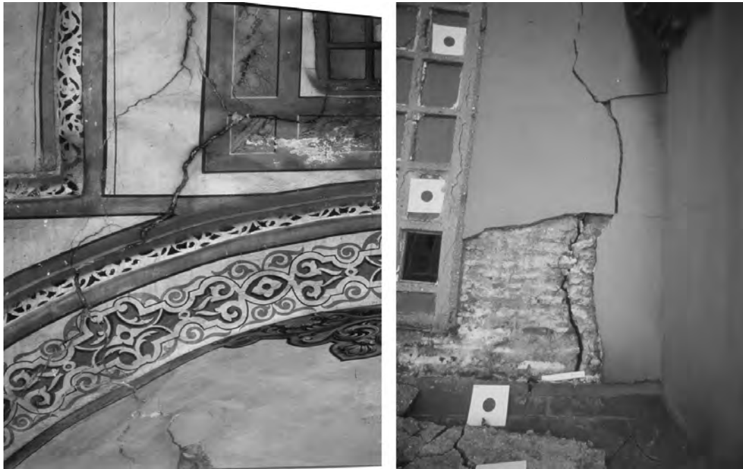
Figure 7 Crack C2 inside and outside after the earthquake from August 17 th , 1999
