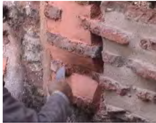
Fig. 5: Application of pozzolanic mortar
