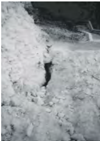
Fig. 4.- Detail of vertical crack in the ground at the toe of the wall
