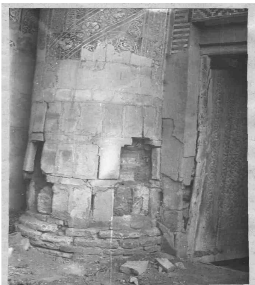
Figure 1. Destruction of the basement of a column as result of lixiviation of salts breaking stability of monuments (Tash-Hauli)
