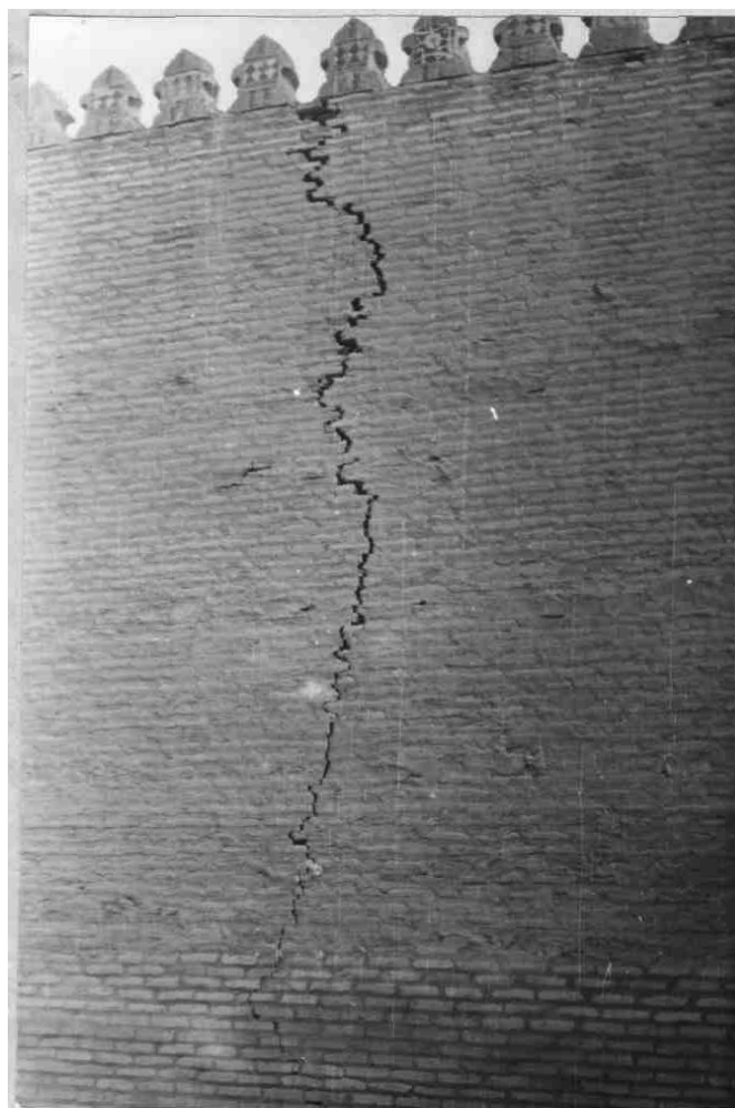
Figure 4. Cracks in the wall of caravan-saray of the complex Alla-Kuli-khan
