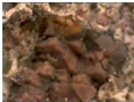
Fig.3 Total loss of binding material. Weathered mortar surface Joints were cleaned by mechanical means and washed out before the pilot application.
