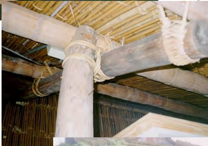
Fig. 3. Column&Purhins Tied by Rattan
