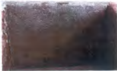
Figure 6.3 Adobe Wall with Cement - Lime Plaster before Rain
