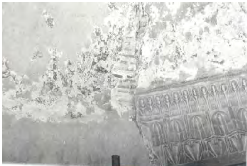
Figure 5. Detachment of the rendering due to moisture at Alkazar
