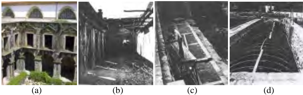
Figure 2 – Aspects of the cloister: (a) present view, (b) demolition of the canon vault, (c) dismounting of the external wall between the large cloister and the small cloister and (d) reconstruction of a reinforced concrete vault
