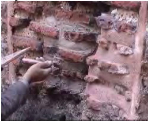
Fig. 4: Application of hydrated lime mortar
