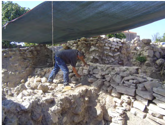
Figure 4: Cleaning of the old mortar
