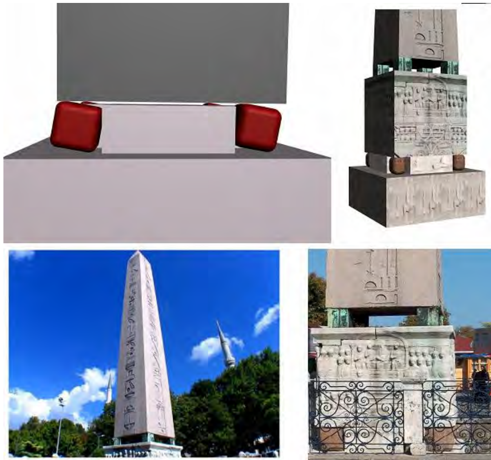
Figure 7: The base isolation of Dikilitas Obelisk
