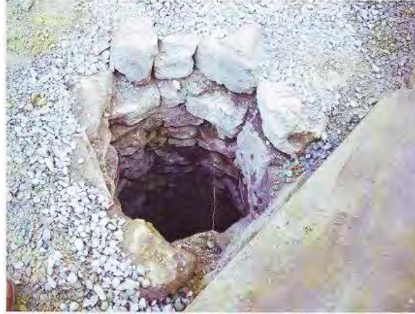
Figure 2: The well of 30 meter deep under the foundation of a two storey small wooden building in Fatih district, Istanbul.
