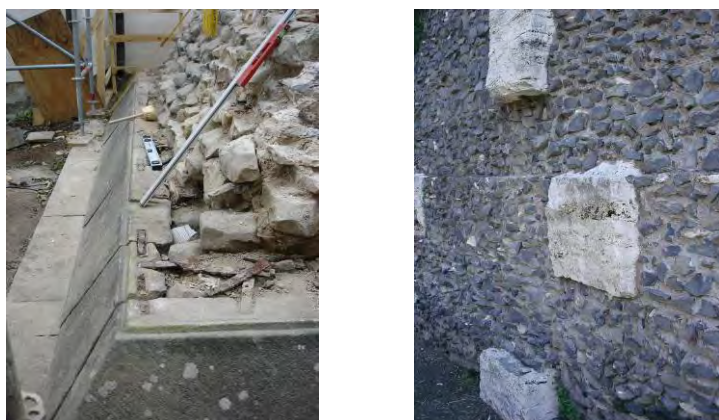
Figure 3: To the left the first course of casing at the Järfälla pyramid with leaded iron cramps along the sides and iron bars running transversely into the concrete core. To the right the base of the tomb of Cecilia Metella at Via Appia with concrete courses with heights corresponding to the remains of the headers. (photos M Traung)
