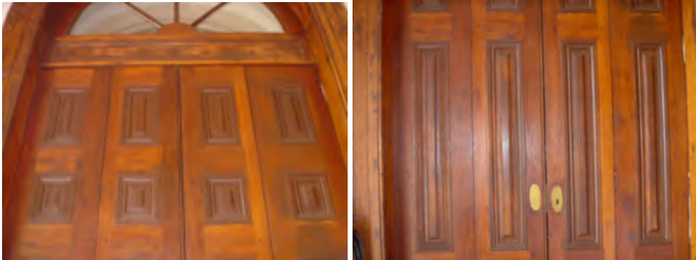
Figure 7: Red Room door: detail of friezes, raised and fielded panels and frames, 2007.
