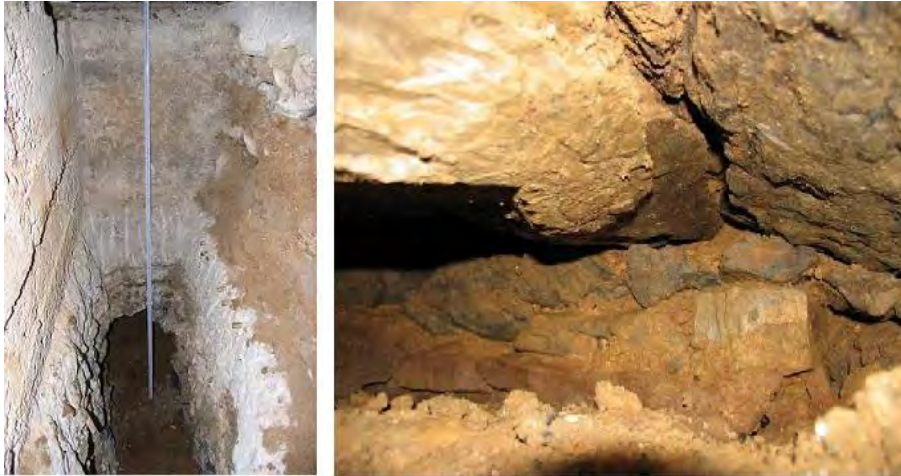
Figure 3: The Galleries or underground gates below the mat foundation (left). The gallery that is filled with soil about 80% during 2 centuries (right)
