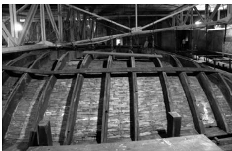
Figure 2. The light mat canes structure nailed an wooden matched and curved centerings which form the characteristic shape of the vault
