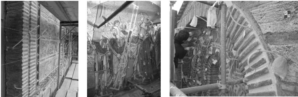
Figure 3: Preparation of the Katholikon masonry and its mosaics before grouting
