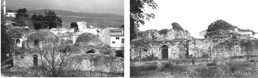
Figures 1a, 1b. Monument before and after the collapse of the soyunmalik dome.
