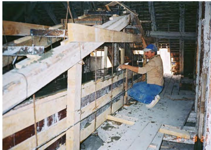
Figure 8 Additional supporting structure of the lifting girder – photo
