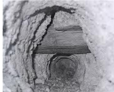
Figure 4: Endoscopy: A sound timber element is disclosed within the wall. Panagia Krina in Chios Island Greece (photo E. Vintzileou)
