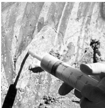
Figure 4 Injection of the plaster from the hole whose sides were reinforced with japanese paper and Paraloid B72 to prevent cracking.
