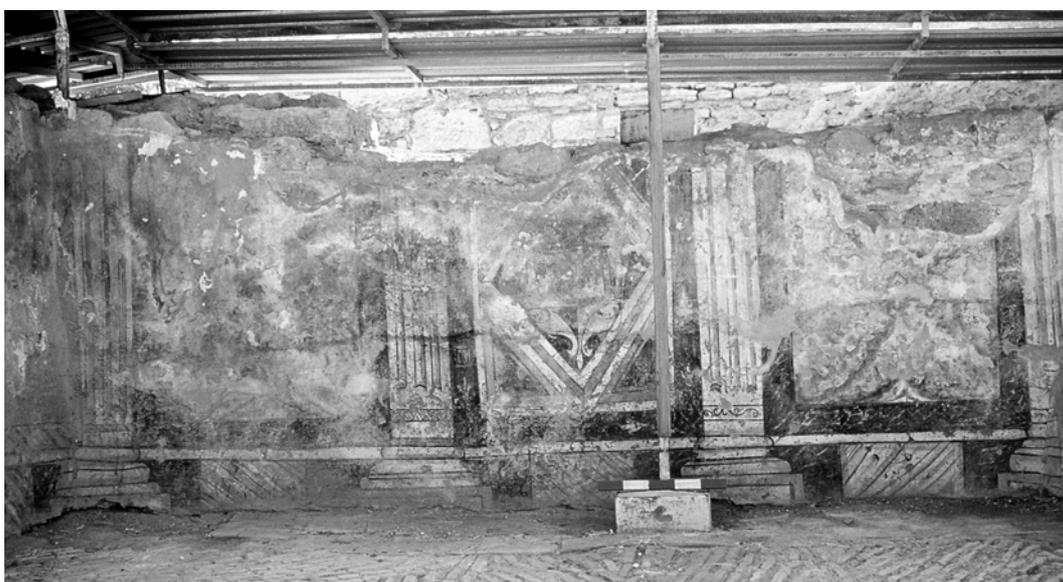
Figure 1 Effloresces hiding the patterns and the colors and the white colored plaster pointings (on the upper part on the left side).
