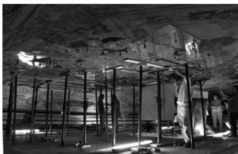
Figure 7. Vault fragments reassembling on cons-shape realized with insertion of stainless steel connectors
