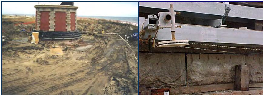
Figure 2 Dewatering around the foundation and cable sawing of the base
