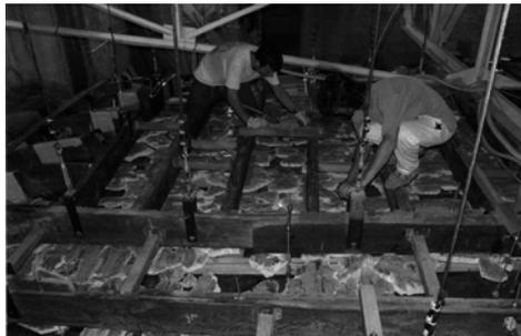
Figure 6. Fragments lay down lean on Plexiglas panels (photo Vassallo)
