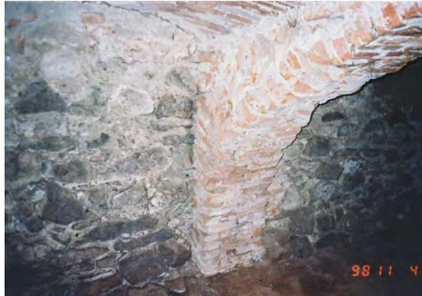
Figure 3 Masonry stone walls, brick arch and vault
