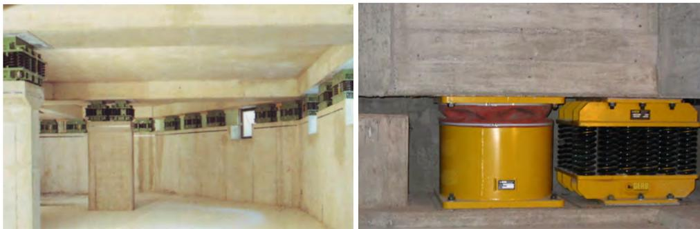
Figure 1 – Elastic Support Systems in Basements of Buildings
