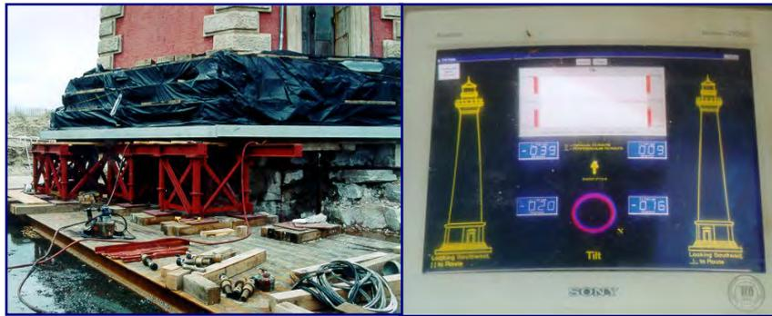
Figure 3 Underpinning of the base and monitoring system against tilt
