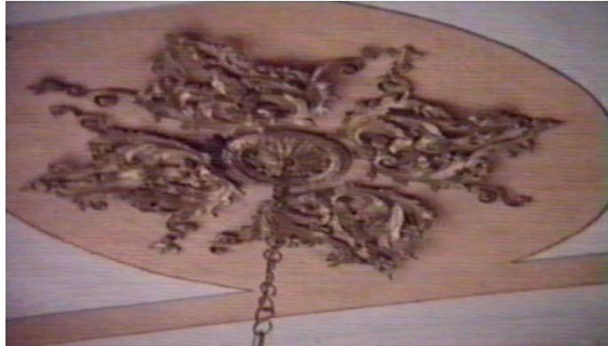
Figure 5 Plastering in stucco of the ceiling
