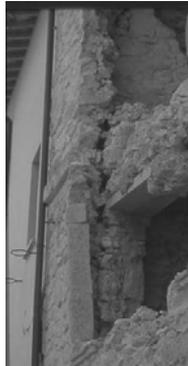
Figure 1. Separation of masonry leaves and collapse under out of plane actions
