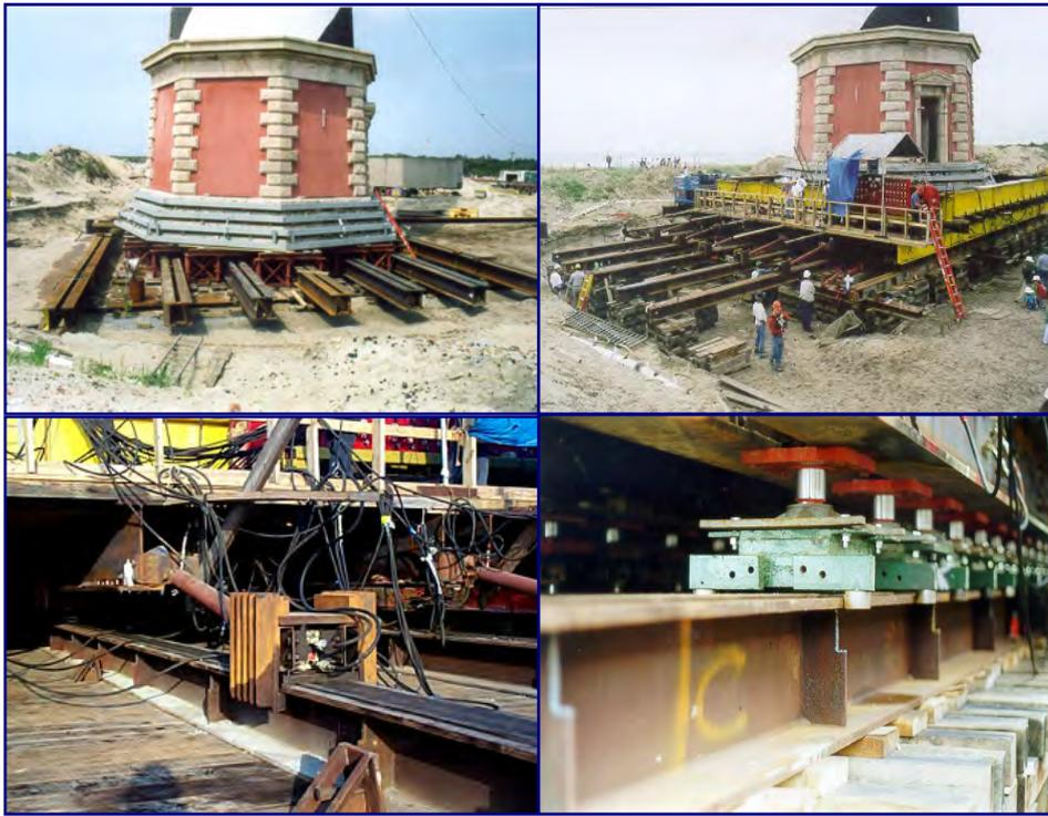
Figure 4 Seven Rails, Support Frame, Jacks and Rollers for the Lighthouse
