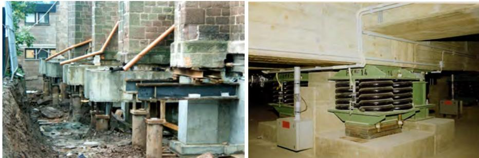
Figure 9 – Structural Upgrade Works and Final Spring Support System
