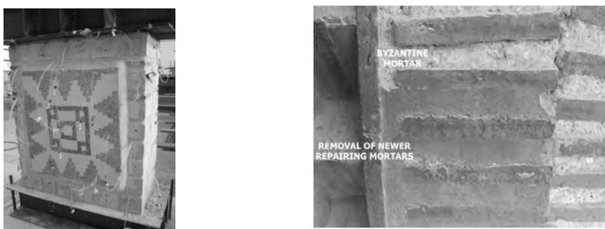
Figure 2: Wallette preparation for grouting (left). Removal of the recent repairing mortars in order to reveal the underlying byzantine mortars of the Katholikon masonry (right)
