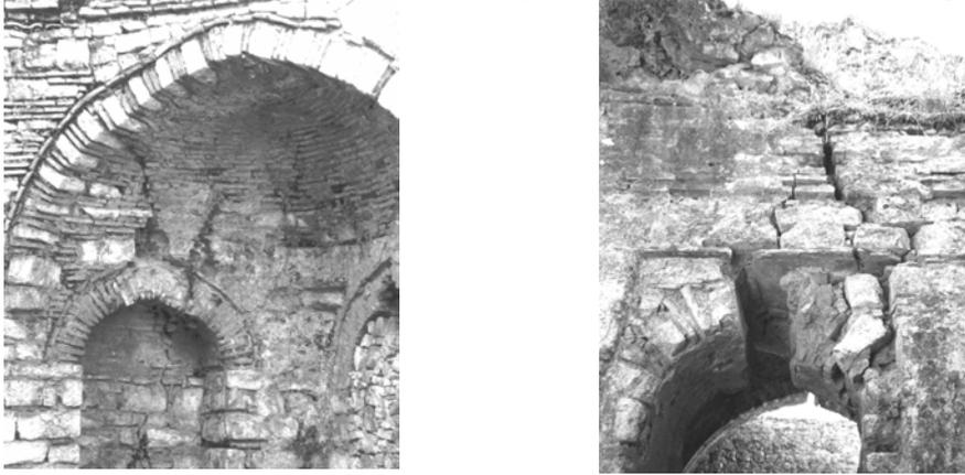
Figures 2a, 2b. Damages at domes and arches.
